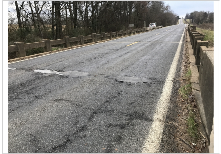
All joints covered with asphalt
