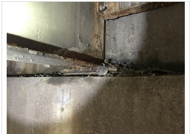
Fixed bearings have heavy pack rust
