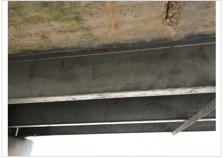
Painted steel I beams
