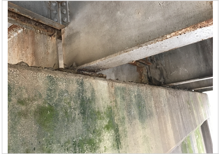
Various beam ends have section loss
